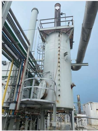
Vertical Cylindrical Radiant Height \approx 18.3' Tube to wall \approx 5.83' Insulation I.D. \approx 6.5'
