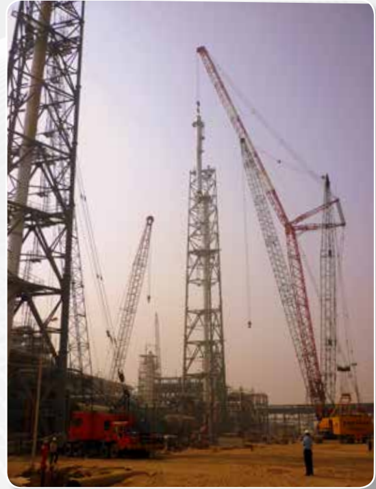
Derrick-Supported Stack Installation
