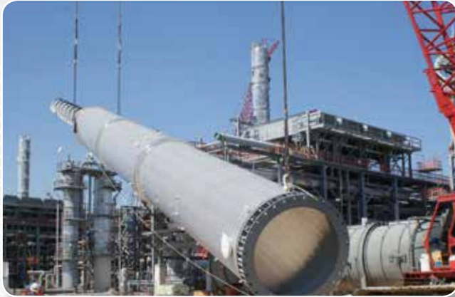
Incinerator Stack Single-Point Lift
